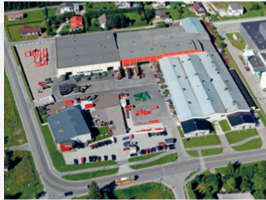
The Fors MW factory is designed for short series production. It is located in Saue, 15 km from Tallinn, Estonia. The production area covers 40,000 m 2 , 18,000 m 2 of which is undercover.
