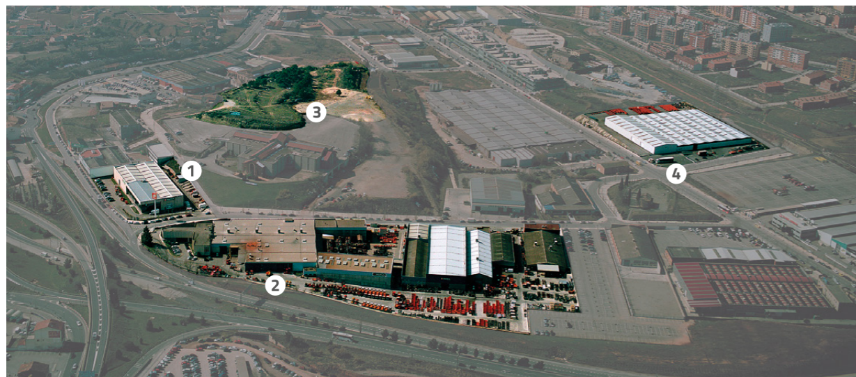
1. Headquarters 2. Assembly plant 3. Test, demonstration and training area 4. Warehouse for completed machines
