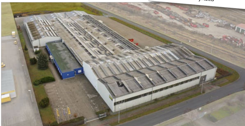
Halberstadt Site II, Manufacturing
