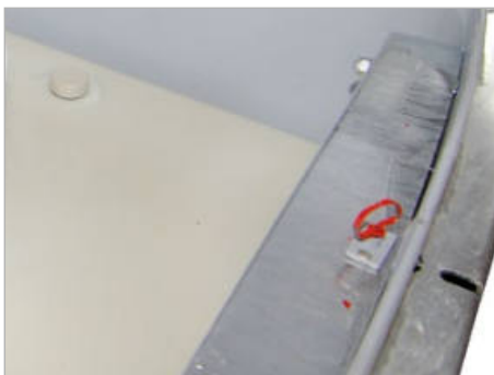
Dipstick to register any leakage
