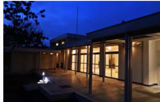
CONSTRUCTION OF THE AUSTRALIAN EMBASSY - RESIDENTIAL AND STAFF AMENITY FACILITIES KABUL, AFGHANISTAN Client: AUSTRALIAN GOVERNMENT DEPARTMENT OF FOREIGN AFFAIRS AND TRADE (DFAT)
