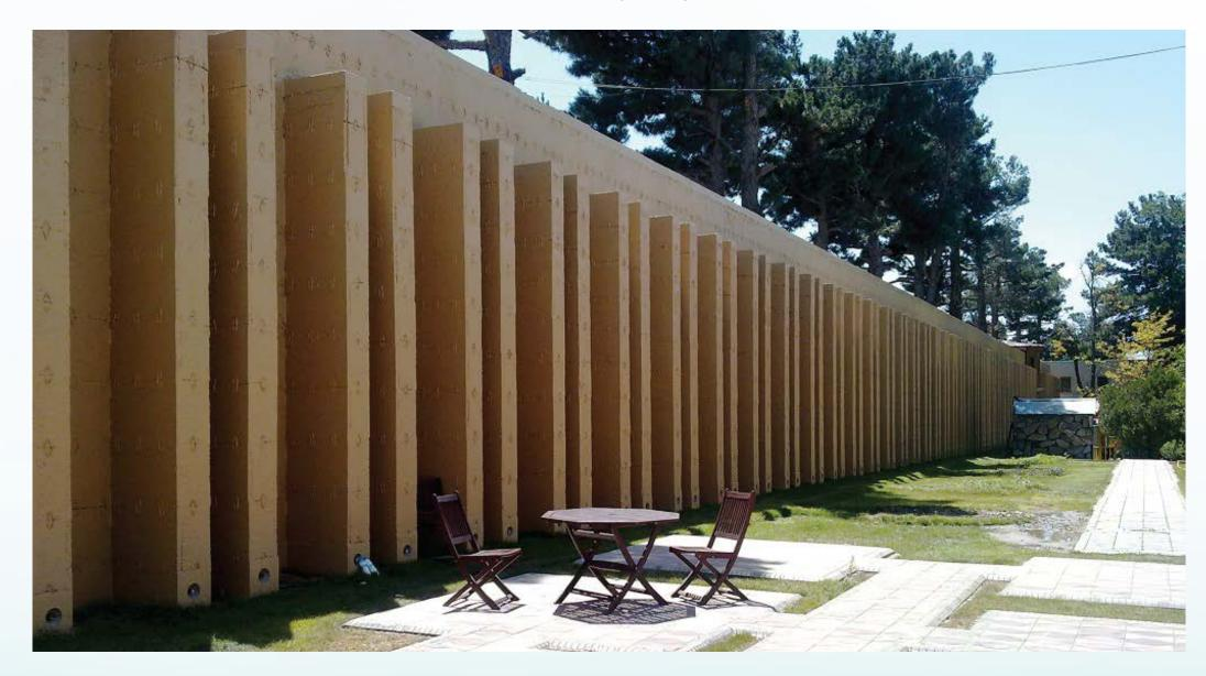
Construction of 1,400 meters long, 7 meters high force protection blast-mitigating perimeter wall and guard towers at ISAF (International Security Assistance Force).
