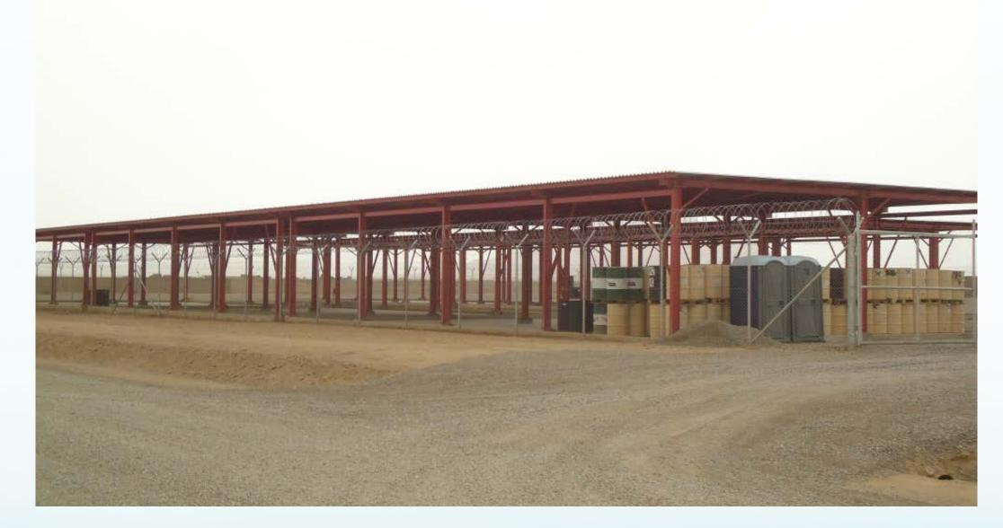
Design and Construct a complete Hazmat Yard including concrete slabs, overhead cover, fence & gates, blast protection, and electric service at Delaram.
