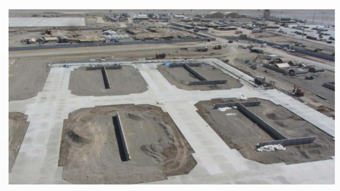
Design and construction of a pavement quality concrete of approximately of 13.000 m<sup>2</sup> for aircrafts including drainage systems, ducting, force protection and markings.
