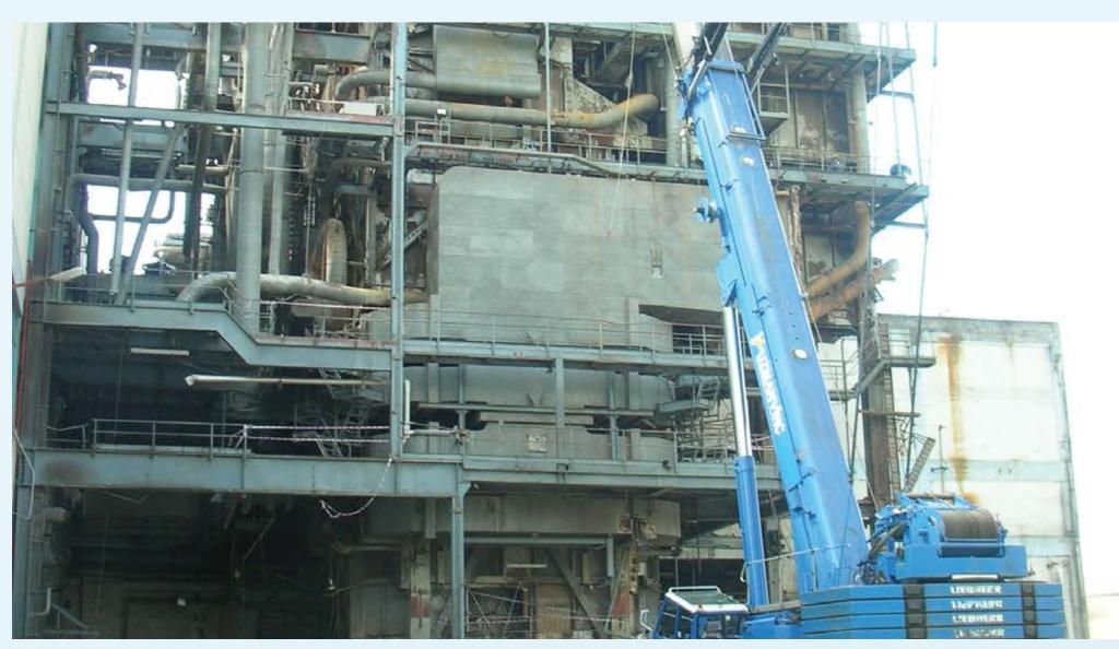
The disassembly and destruction of the Ambarlı Fuel-oil power plant units number 4 and 5 having a capacity of 630 Megawatt together. Dismantling of 8.000 tons of structural steel, equipment and pipe, destruction of 5.000 tons of brick wall and bread down of a 102 meter height gas stack are under our subsidiary company Mak-in's responsibility in 3 months.
