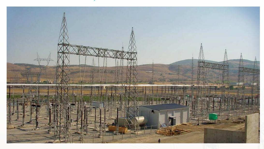
Design & Construction of 380kV Switchyard including Civil Works (excavation, foundations, trenches, control bldg, earthing, steel structures) and Electrical Works (primary equipment installations, protection & control system, RTU & Telecommunication System, AC/DC Auxiliaries, cabling, lighting, lighting protection, testing & commissioning etc.
