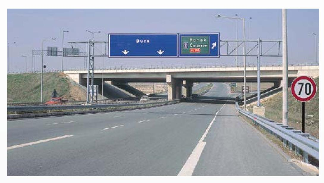
The project scope consists of the rehabilitation of super structure; construction of asphalt concrete binder and wearing layers for 109 km section of Izmir-Aydın-Çeşme motorway and branches. Earthworks: 89,500 m<sup>3</sup>; 6cm compacted thickness asphalt concrete binder: 395,650 m<sup>2</sup>; 5cm compacted thickness asphalt concrete wearing layer: 3,742,000 m<sup>2</sup>; road marking and signs
