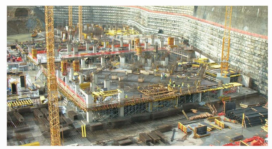
Civil works construction of shopping mall, Car Park, Office, Residence total amount of 520.000 m<sup>2</sup> formwork, 155.000 m<sup>3</sup> concrete, 30.412 tons of rebar by our subsidiary company Mak-in.
