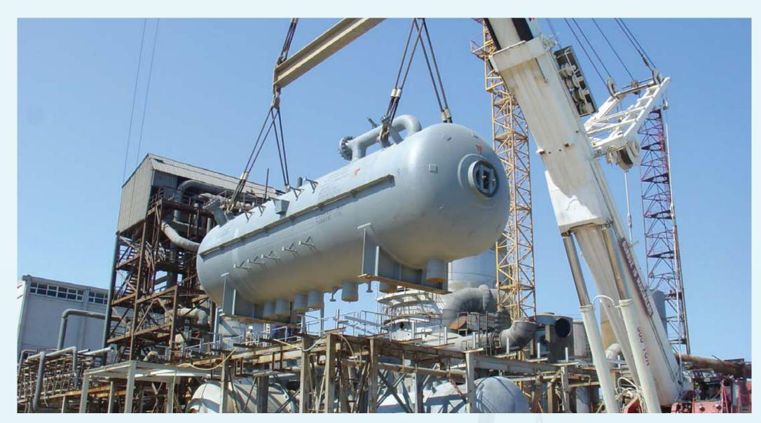
Renovation works for the Suplhuric Acid Plant with the total amount of 4,500 tons of Carbon steel, stainless steel equipments and manufacturing machineries. The Assembly works were completed in a record of 4 months at Turkey's largest Sulphuric Acid Plant by our subsidiary company Mak-in.
