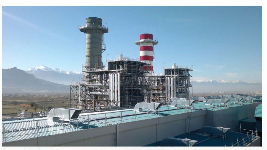
All civil works, architectural works and major parts of steel works and equipment assembly works for a 800 MW Combined Cycle Power Plant by our subsidiary company Mak-in.
