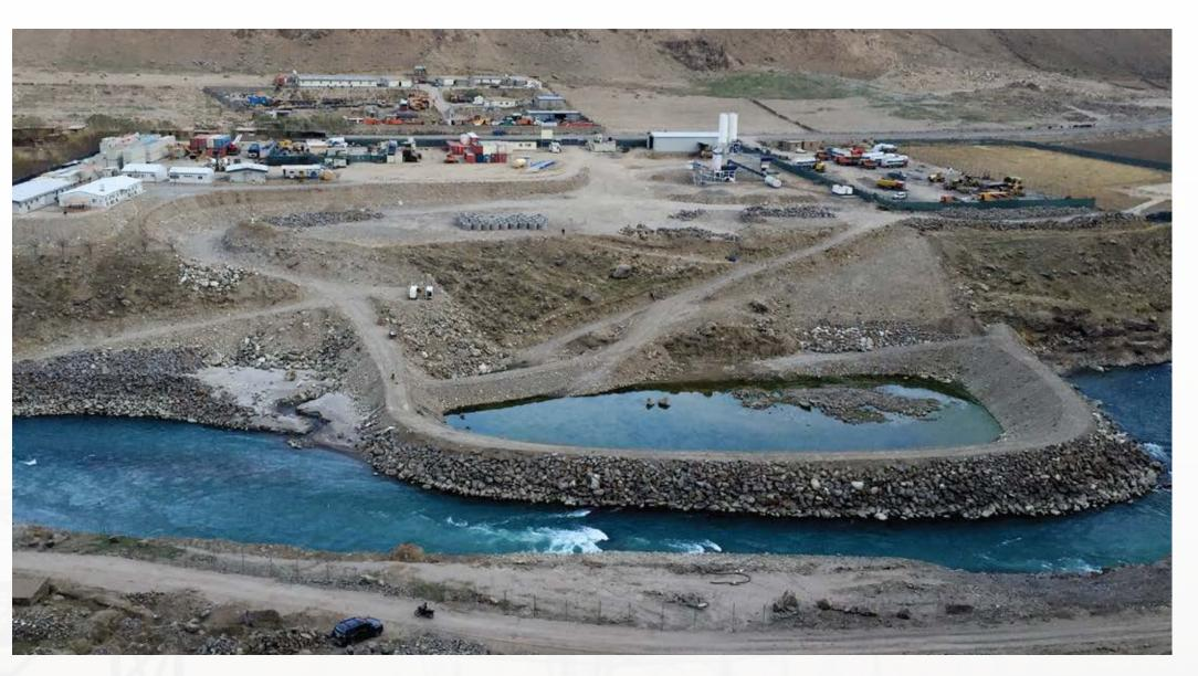
Design and build contract for a turnkey construction of 7,6 MW Hydro Power Plant (3 x 2,54MW - Vertical Axis Kaplan-Type ). All Civil Works, Hydraulic Steel Structures, Electromechanical Equipments, Electrical Balance of Plant, Mechanical Balance of Plant.
