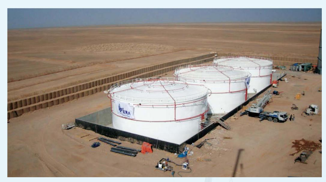
Construction of 6 each Jet Fuel Steel Tanks with total capacity of 30 million liters, 8km 6"jet fuel pipeline.
