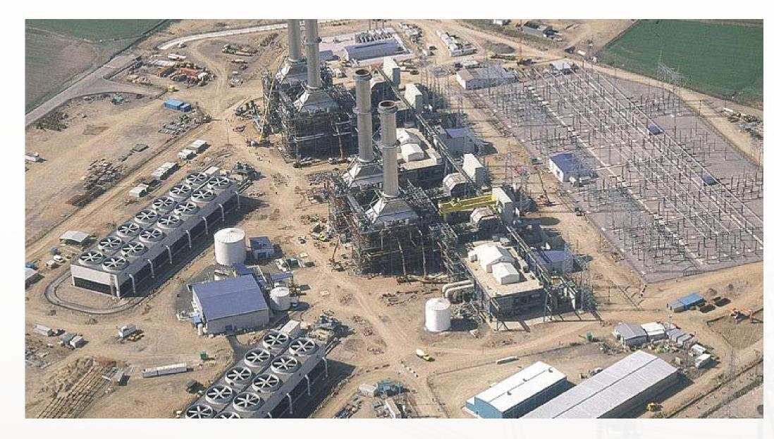
Civil works of cooling towers, switchyard, construction of salt field, infrastructure and earth works, BOP construction works (water treatment building, pre-treatment unit, pipe racks, filter, slurry thickeners, slurry sump, fire/filtration water tank, neutralizing tank, potable water tank, clear well tank, sodium hypo-chloride unit, chemical waste sump, valve room etc.), earthing, site civil works and perimeter fencing
