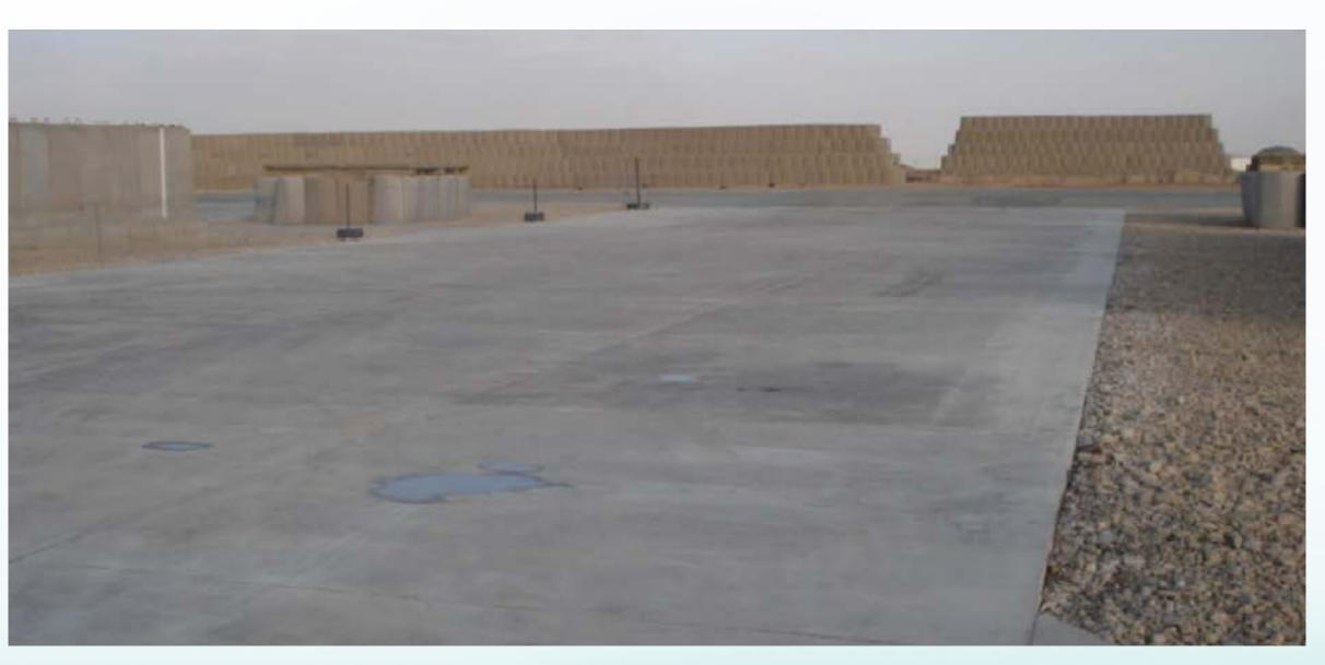
The project consists of removal, cleaning of approx. 10,030 m<sup>2</sup> matting, construction of 43,300 m<sup>2</sup>, 25 cm in thickness of un-reinforced Pavement Quality Concrete (PQC), construction of 300 m HESCO walls, 400 m road, drainage system, painting of taxiway lines and installation of aircraft earthling points.
