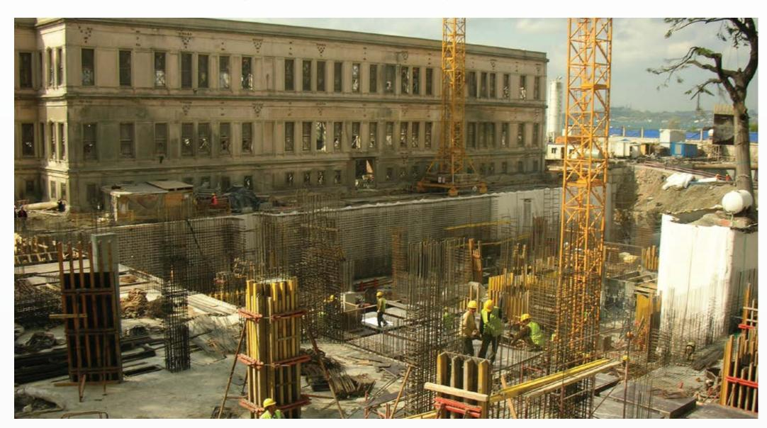
Construction of civil works for a five star hotel with total amount of 97.000 m<sup>2</sup> form work, 35.700 m<sup>3</sup> concrete, 3.950 tons of rebar by our subsidiary company Mak-in.
