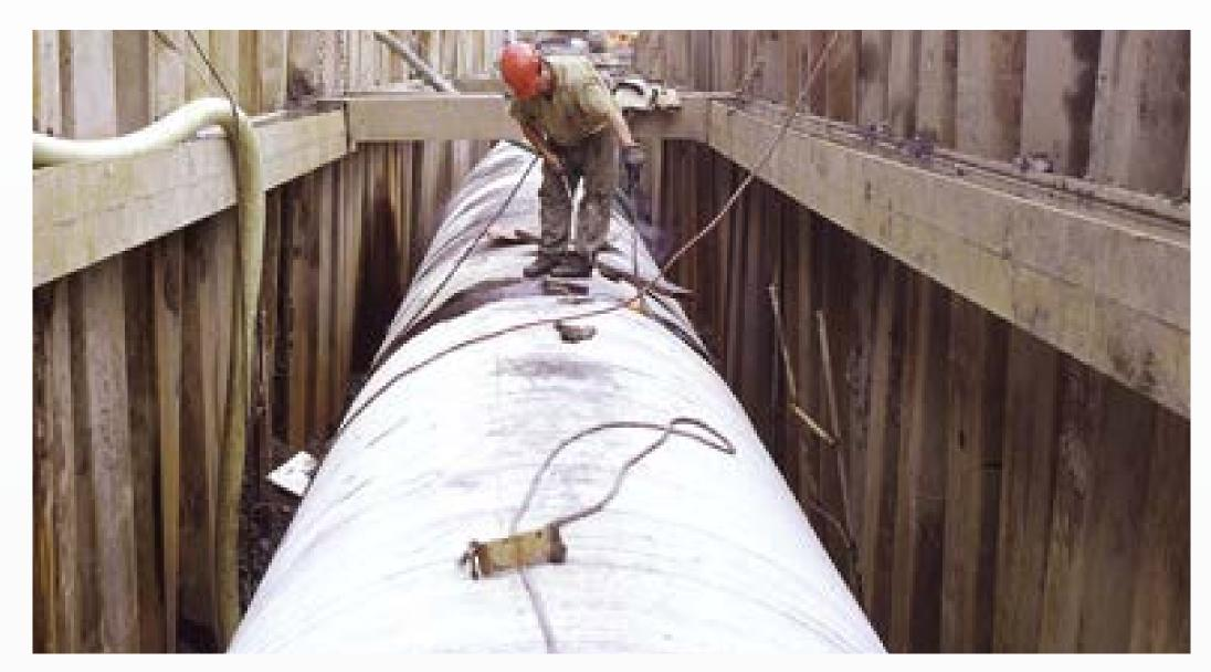
Excavation of trench, 3.880m reinforced concrete pipe laying, backfilling and compaction, displacement of existing underground utility lines, repair of roads and asphalt pavement
