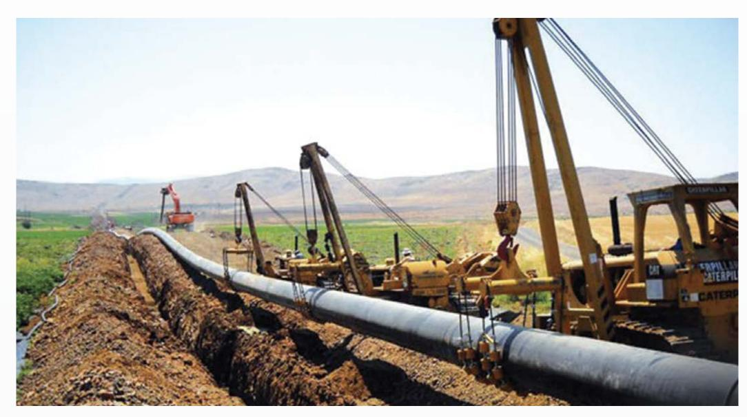
Construction of 106.9 km, 12" PN 100 fuel pipeline,10 line valve pits, 4420 m river crossing.
