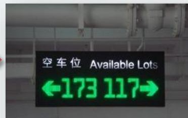
In Parking guidance signage
