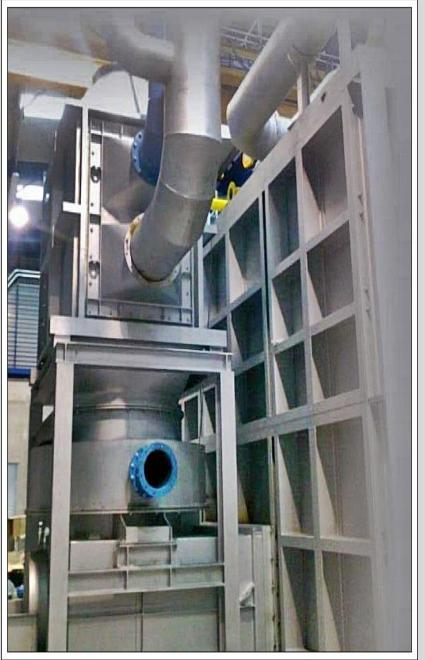
The combustion system with cold air setting pulses allows the optimization of combustion, obtaining one of the best effects of heat exchange.
