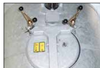
Ø 600 mm upper manhole on hinge
