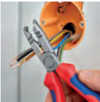
Cutting when shortening single conductors
