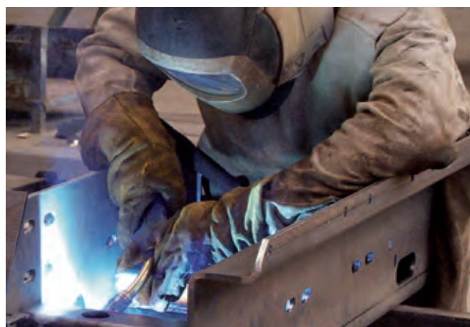
Welding a welded assembly to the frame.
