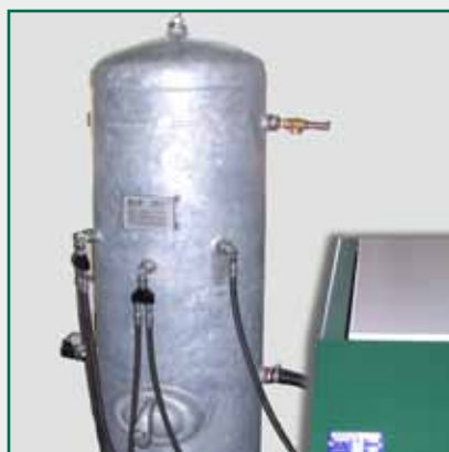
150 l primary pressure tank for condensate return
