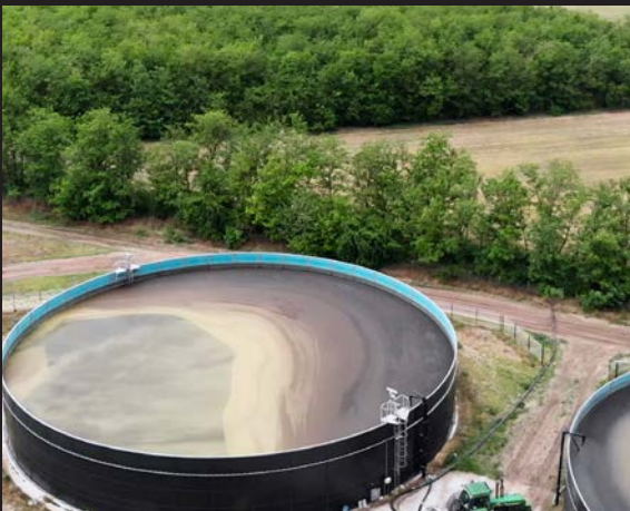
SLURRY TRANSFER IRRIGATION LINE
