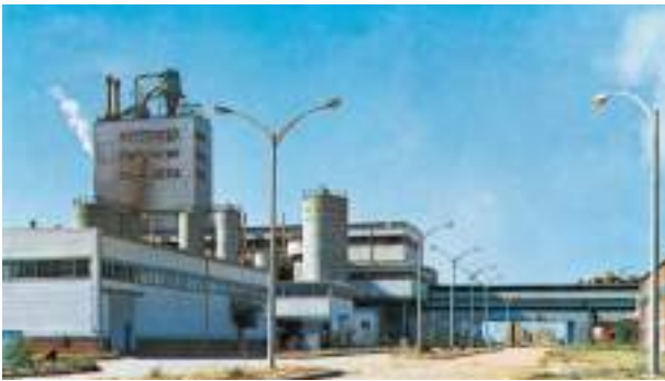
Çay Cellulose Facilities, Afyon/Turkey Çay Selüloz Tesisleri, Afyon
