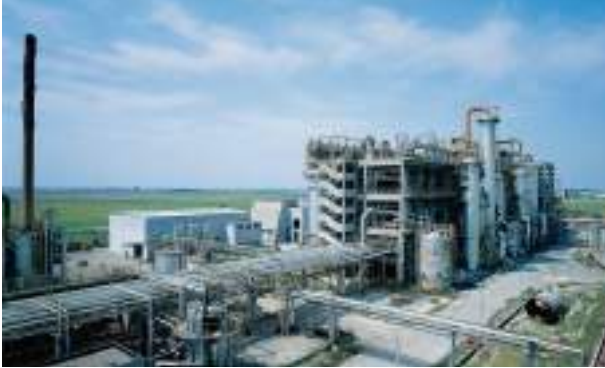
SASA DMT Plant and Facilities, Adana/Turkey SASA DMT Fabrika ve Tesisleri, Adana
