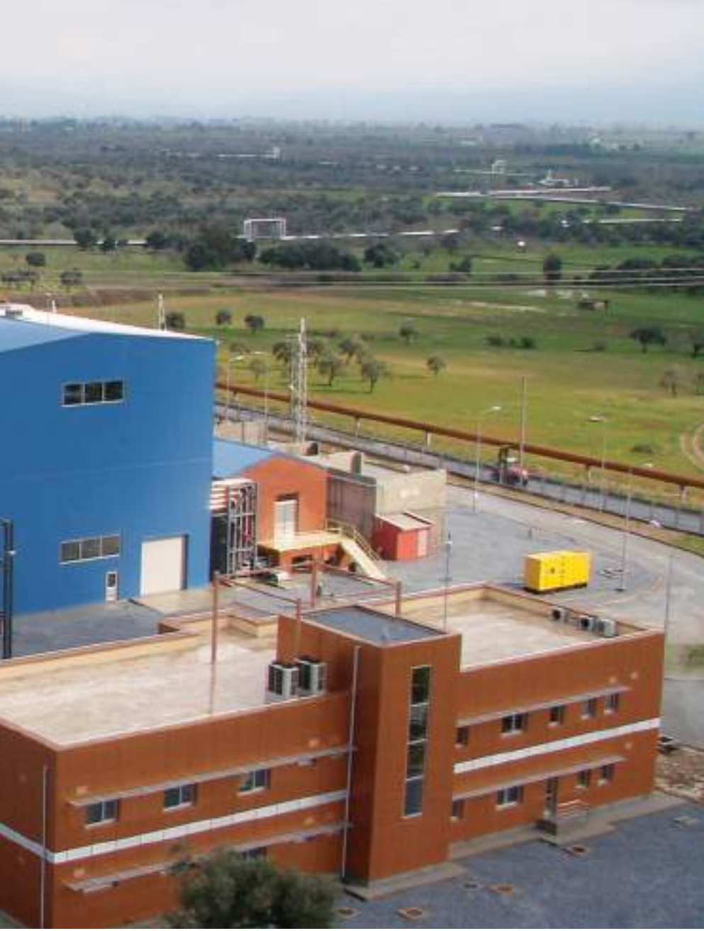
47,4 MW Galip Hoca Geothermal Power Plant Project, Aydın/Turkey
