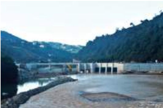
16,35 MW Arca Hydroelectric Power Plant, Trabzon/Turkey 16,35 MW Arca Hidroelektrik Santrali, Trabzon
