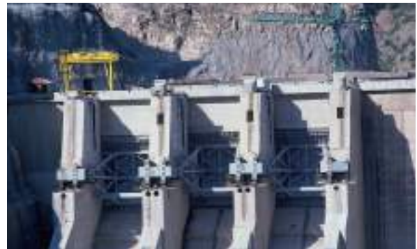
SIR Dam and HEPP, Manufacturing and Erection of Hydromechanical Equipment, Kahramanmaraş/Turkey SIR Barajı ve HES Tesisleri, Hidromekanik Ekipman İmalat ve Montajı Kahramanmaraş
