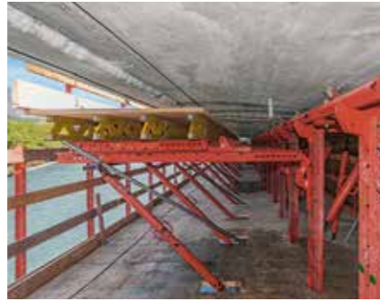
The moveable units were attached via rollers and rails completely to the underside of the cantilever which meant the superstructure remained freely accessible.
