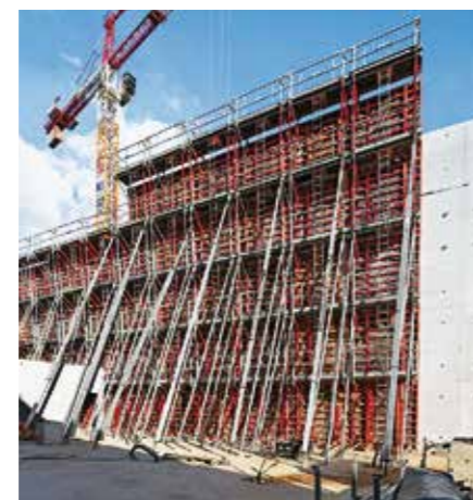
Modular safety: the MXP Platform System exactly matches the element widths of the MAXIMO and TRIO Panel Formwork Systems.
