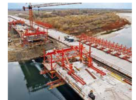
The Balanced Cantilever Equipment can be flexibly adapted to suit diverse superstructure geometries; traffic flow is not affected.
