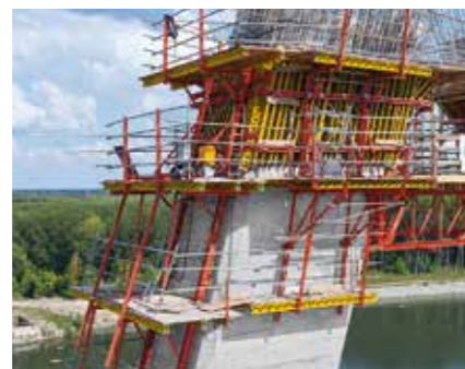
RCS, CB and VARIO GT 24 formed the ideal climbing combination for constructing the two bridge pylons.
