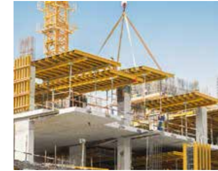
The project-specific planning facilitates very cost-effective slab tables as the static load of the individual components is optimized.
