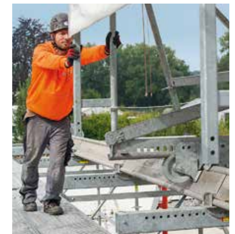
The roof elements can be moved in the longitudinal direction by means of wheels so that, for example, materials can be lifted in by crane.
