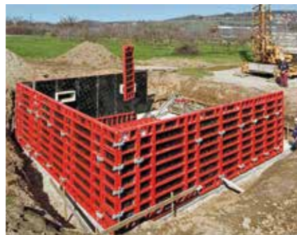
A minimum of different components facilitate easy and fast forming with TRIO – both in single-family housing construction as well as for large projects.
