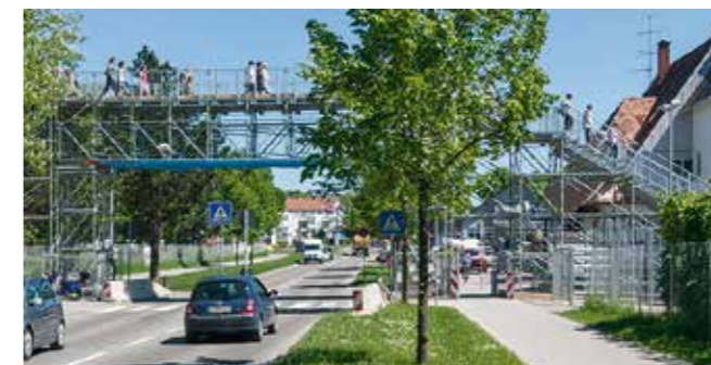
LGS is suitable for temporary pedestrian bridges and meets the requirements regarding guardrail loads and geometries for use in public areas.
