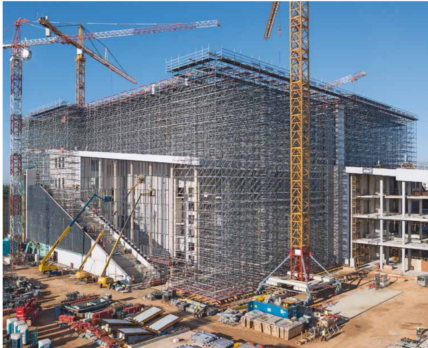
For earthquake-resistant implementation, PERI UP was supported on a load-distributing VARIOKIT construction.
