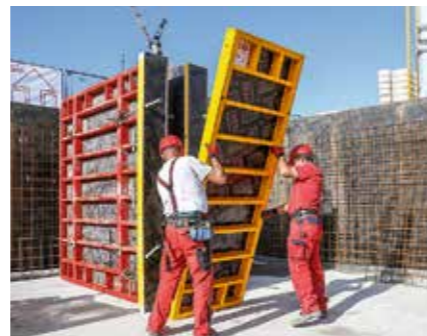
The aluminium TRIO panel elements are yellow powder-coated; they can easily be moved by hand.
