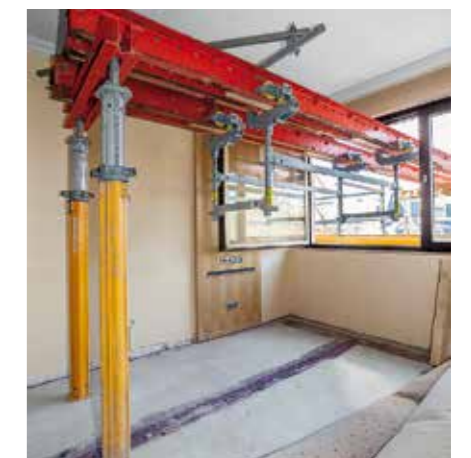
Using RCS Rails and Trolleys from the PERI UP System allowed bulky components to be easily moved through the window openings to the outside.
