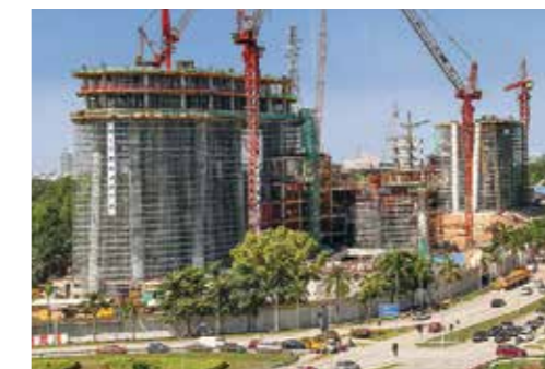
Above, slab tables on a PD 8 basis served for forming the floor slabs; below, PERI UP ensured a safe transfer of loads.
