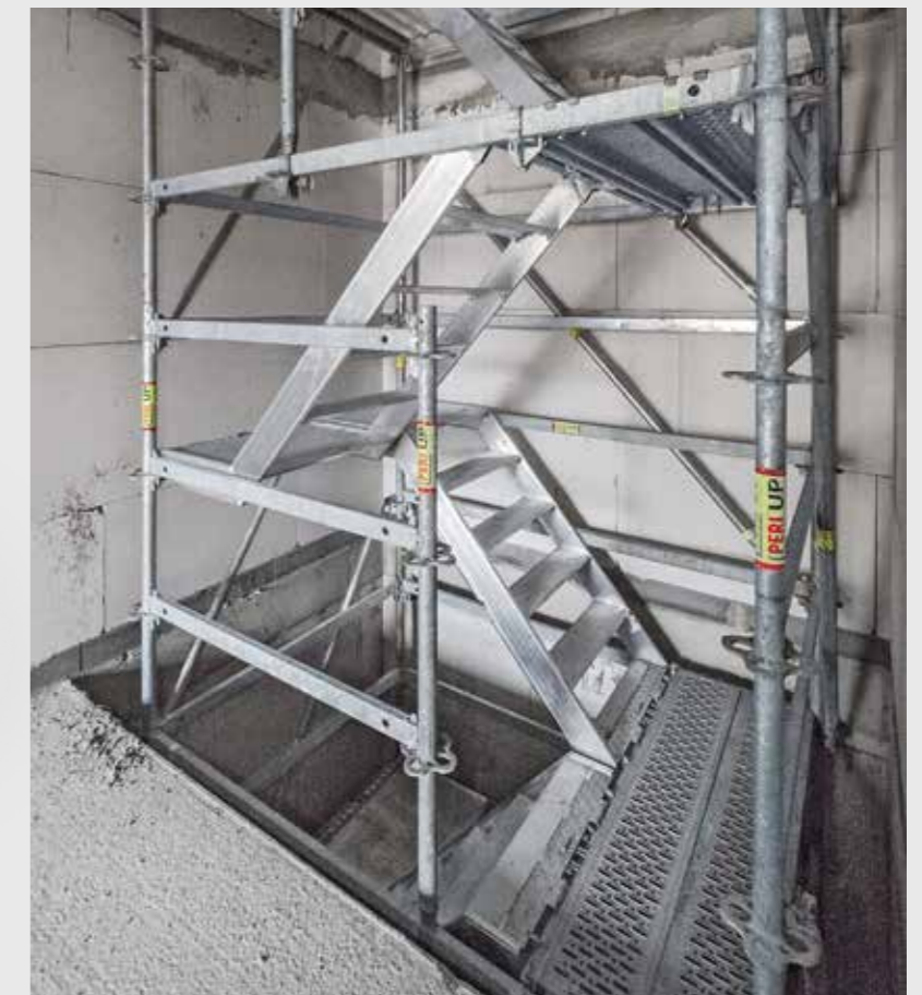
Height adjustments to building openings are carried out by means of short flights of stairs and externally mounted brackets – regardless of the floor height.
