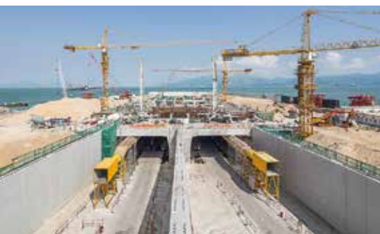
300 m long ramp structures with high walls in architectural concrete quality serve as the entrance and exit points of the 6 km long HZMB tunnel.
