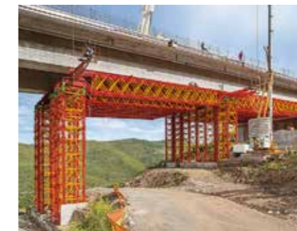
VARIOKIT Heavy-Duty Shoring Towers and Truss Girders serve as load-bearing falsework for the edge sections of a 412 m long motorway bridge.
