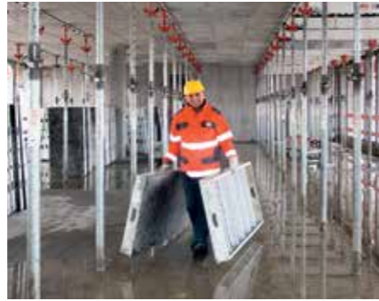
The approx. 15 kg lightweight system components support quick and simple working operations with SKYDECK.
