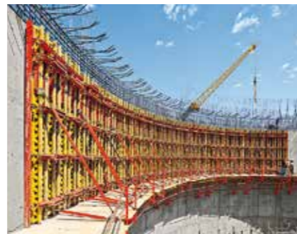
The radii of the RUNDFLEX panels are adjusted with spindles. Adapting to changing radii is therefore carried out extremely quickly.
