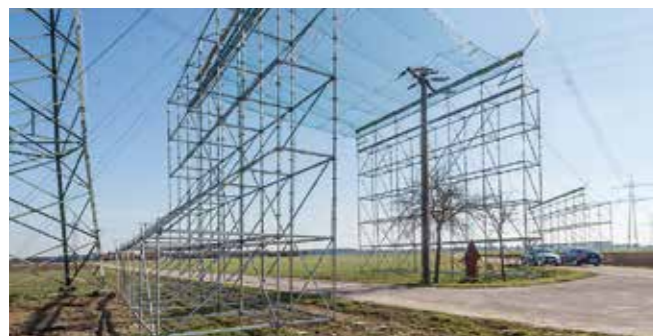
For work carried out on overhead lines, PERI UP protection scaffold comprised of lightweight system components secured the crossings over the public roads.
