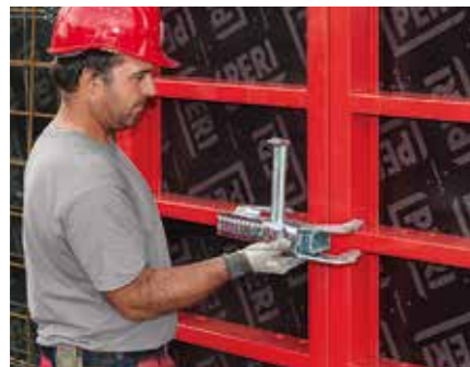
The BFD Coupler can be operated with one hand. The framed panels are connected flush, aligned and tight in one working step.
