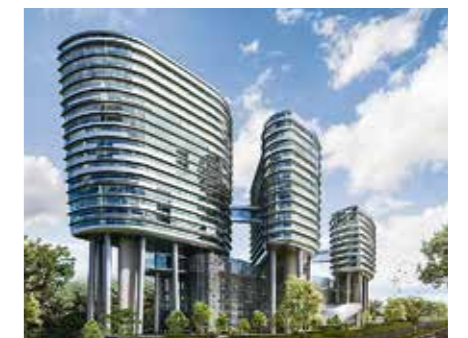
Three elevated high-rise structures form the new SPRM administrative centre (Suruhanjaya Pencegahan Rasuah Malaysia); model image: Mitrajaya Holdings Bhd.
