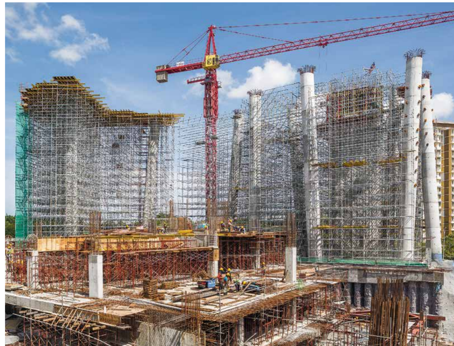
Working scaffold, bracing and shoring rolled into one: PERI UP subsequently followed as birdcage scaffolding within the cycle of the RCS Climbing Formwork.
