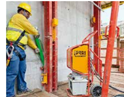
The mobile climbing device allows climbing without a crane. The hydraulic cylinders are mounted on the climbing shoe between the wall and climbing rail.
