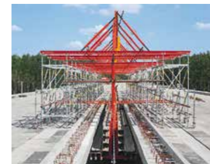
By means of simple rollers, the formwork and supporting construction could be quickly moved as one unit to the next concreting section.
