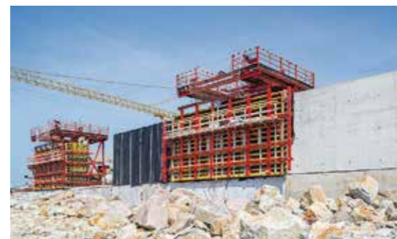
Also for the massive breakwater, the construction team used a mobile wall formwork solution.
