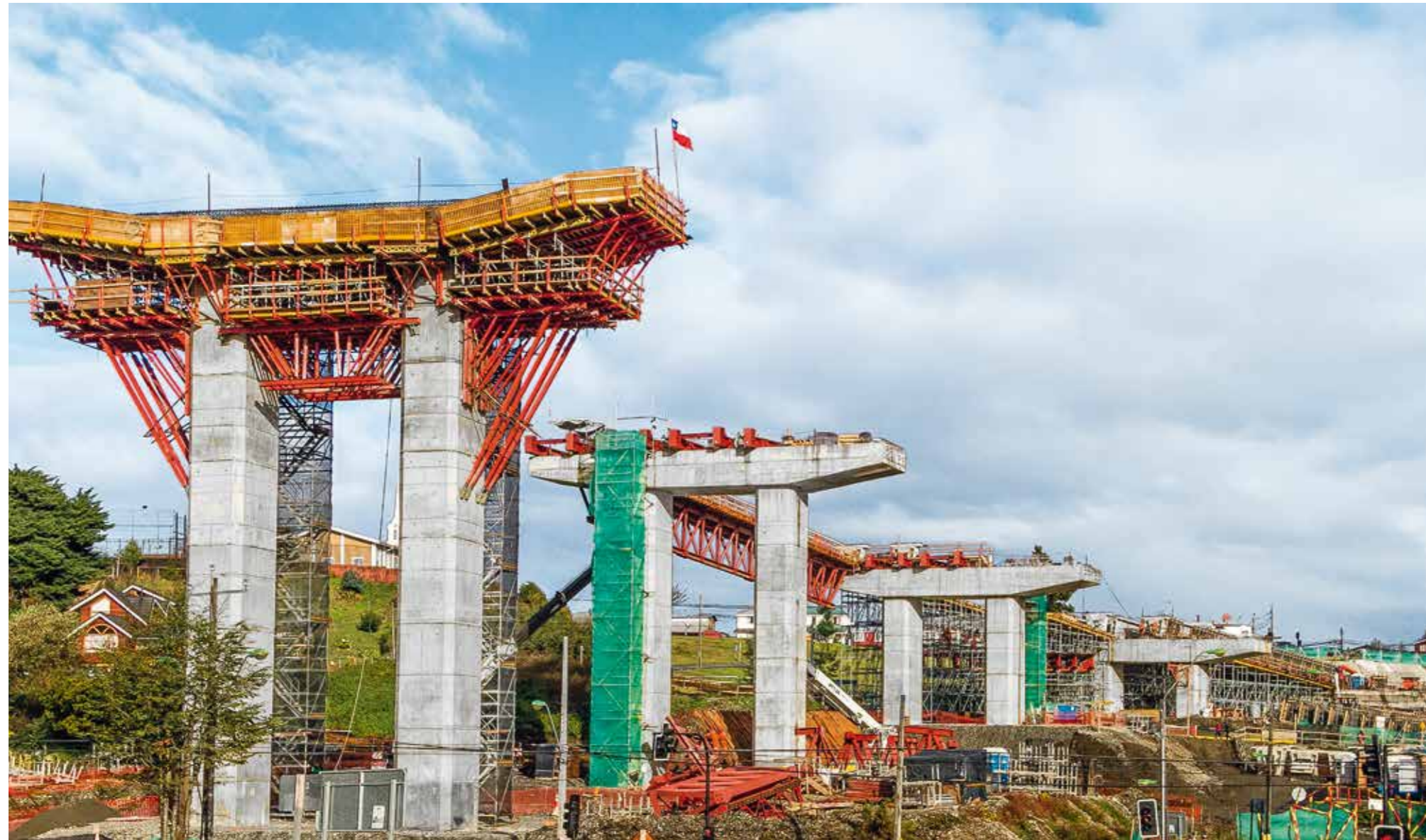
Customized system combination: above the VARIOKIT construction, PERI UP served as a shape-providing load-bearing system. TRIO Panel Formwork was used as side formwork while PROKIT Side Mesh Barriers mounted end-to-end provided a high level of safety when working at great heights.
