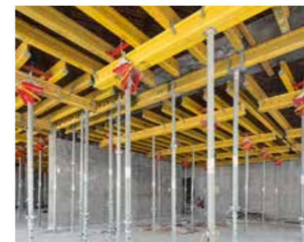
Slab tables with the integrated Table Swivel Head and PEP Ergo Slab Props are an integral part of the comprehensive PERI complete solution.
