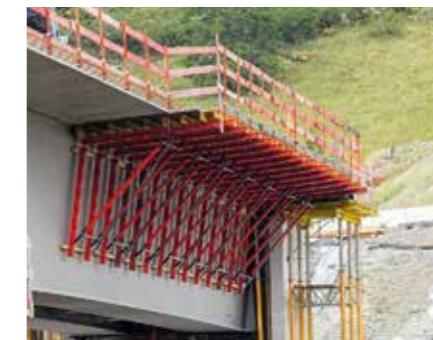
The Cantilever Bracket is used in steel composite or precast concrete bridges in order to concrete the edge areas of the bridge superstructure.
