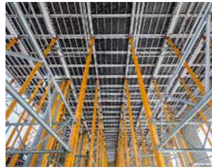
Lightweight and flexible SKYDECK and MULTIPROP System Components made of aluminium saved both time and money when forming the storey slabs.
