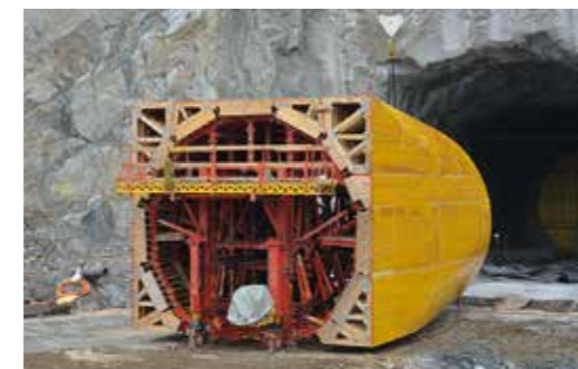
Dimensionally-accurate prefabricated formwork elements allowed the transition from circular to square-shaped tunnel cross-sections.
