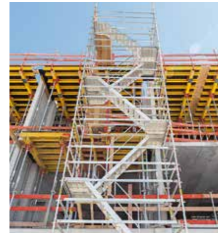
With the Stair 75, all working levels on construction sites can be quickly and safely reached.
