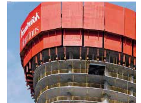
The Climbing Protection Panel can be used in a line also with protruding and recessed slab edges. For this, the supporting components are used together with horizontal RCS Climbing Rails.
