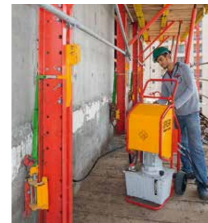
Mobile RCS hydraulic aggregates and cylinders reduced the cost expenditure for crane-independent climbing.
