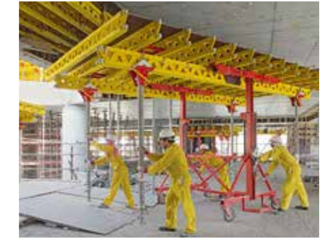
For large slab thicknesses and high loads, high load-bearing GT 24 Formwork Girders are used.
