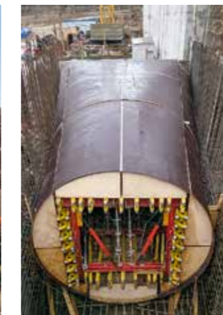
The 3D tunnel formwork construction on a VARIOKIT system basis allowed the dimensionally-accurate realization of the transition from square-shaped to circular discharge structure cross-sections.
