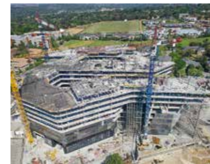
The new Sasol headquarters has seven basement and ten upper floors with a total of 202.000 m 2 .
