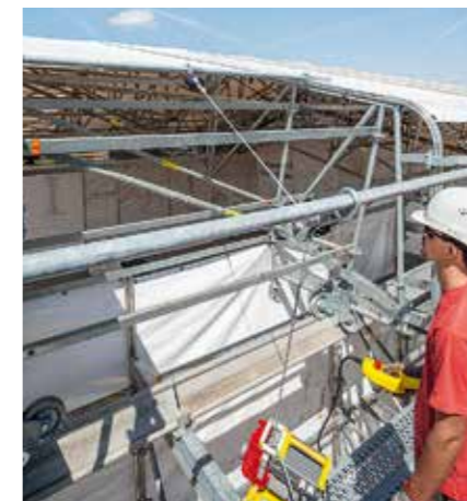
As an option, the tarpaulin can be closed by means of an electric drawing-in device. One tube facilitates the drawing in of the Keder rails.
