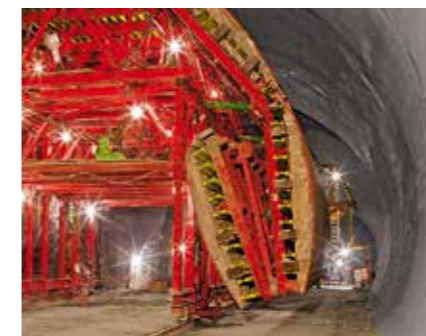
For moving the formwork carriage through a narrower cross-section, the formwork segments can be hydraulically folded.
