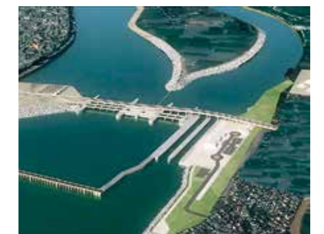
The new Nile barrage is used for water regulation and electricity generation; for ensuring smooth shipping operations, a 120 m long double sluice bridges the 4 m difference in height.
