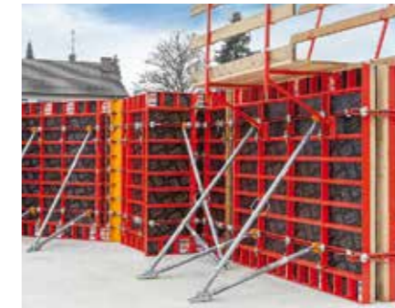
Push-Pull Props and Kickers are attached to the anchor struts of the panel by means of the LIWA Brace Connector.
