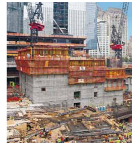
For the external walls of this 47 m x 43 m building core, the ACS R variant provides the optimum solution.
