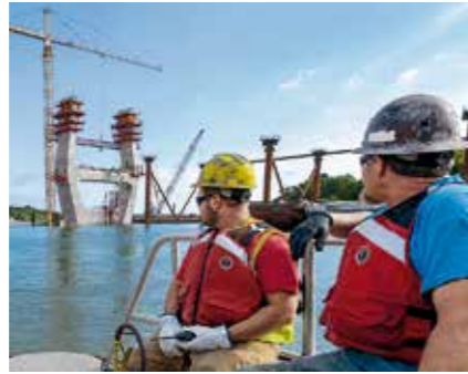
Continuous construction support and a competent planning service: the catwalk featured between the two pylon legs was also an integral part of the PERI complete solution.
