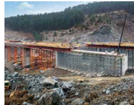
VARIOKIT Engineering Construction Kit: the head spindles of the 4-legged VST Heavy-Duty Shoring Towers could also be operated when fully loaded by means of mobile hydraulics. In addition, the modular system allowed modifications to take place on the bridge piers as well as the use as 2-legged main beam frame.
