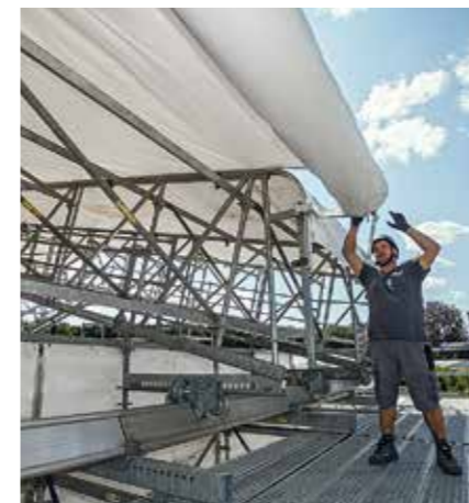
Smooth-running rollers support the uniform rolling up procedure and fast dismantling of the Keder tarpaulin across the entire field width.
