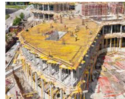
MULTIFLEX can be adapted to suit all ground plans. The overlapping of the slab girders and change of direction of the main beams ensure maximum flexibility.
