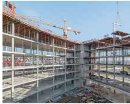
The VARIODECK Table provides a quick and safe solution for slab edge areas in particular.
