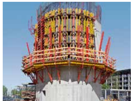
The use of RUNDFLEX on climbing brackets during the construction of a bridge.
