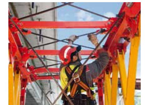
Bolted connections reduce assembly time during installation. The centric bracing connection ensures a high load-bearing capacity.
