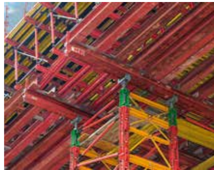
VARIOKIT Engineering Construction Kit: the head spindles of the 4-legged VST Heavy-Duty Shoring Towers could also be operated when fully loaded by means of mobile hydraulics. In addition, the modular system allowed modifications to take place on the bridge piers as well as the use as 2-legged main beam frame.
