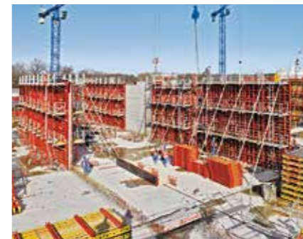
The platform system, consisting of working platforms, access ladders and guardrails, provides maximum safety.
