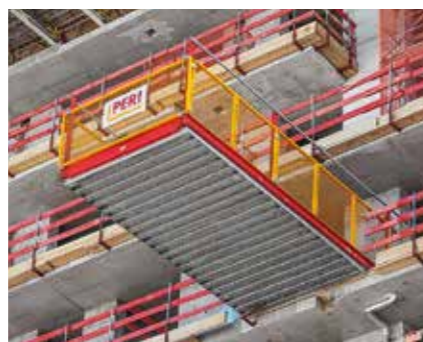
The RCS MP Platform complete with steel decking for moving materials is available as standard in two sizes.
