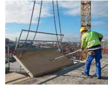
The SKYDECK platform ensures safe working conditions at the slab edges and saves the installation of safety scaffold in the level below.
