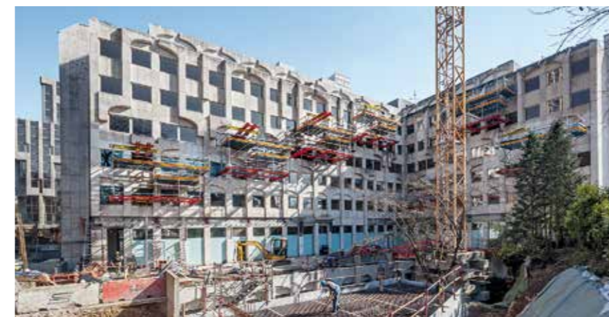
At the same time as the construction measures on the ground floor, the 165 hotel rooms in the floors above were completely refurbished with the help of cantilevered PERI Platforms.
