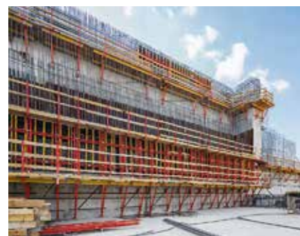
VARIO Formwork, CB Climbing Platforms and PERI UP access technology guarantee easy handling along with a high level of safety.
