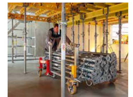
With the easy to use pallet wheels, materials can be quickly moved by hand to the next place of use.
