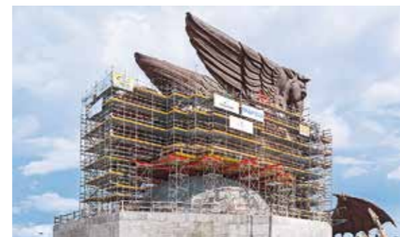
VARIOKIT System Components supplemented the PERI UP Scaffold Solution in particular for the large-span bridging.
