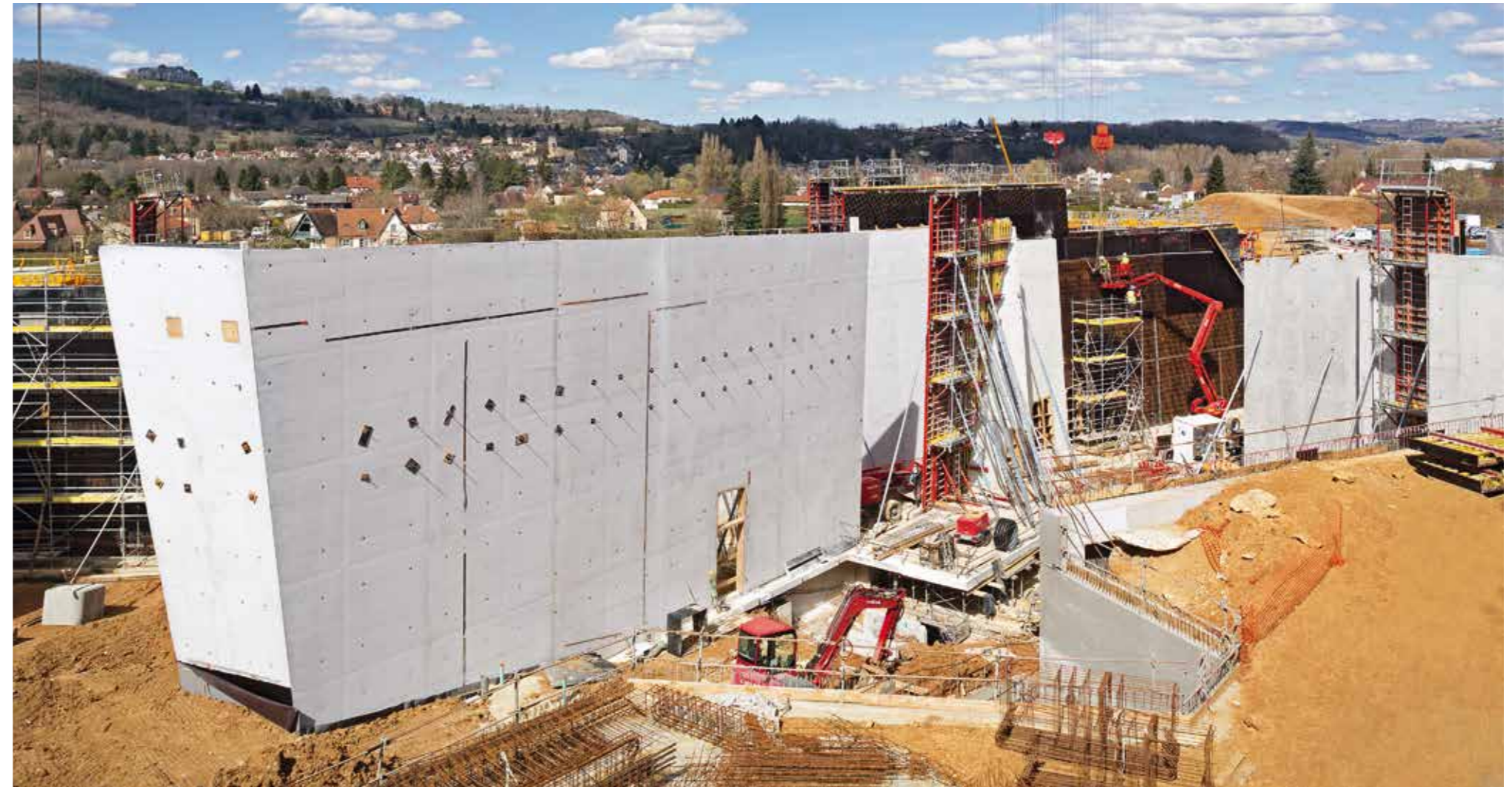
The MXP Platforms are securely connected with the TRIO components. With only a single crane lift, complete large-area units could be moved.
