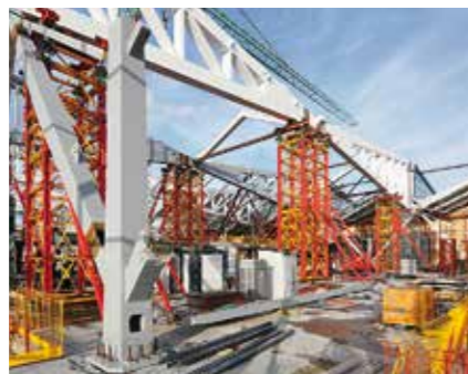
VARIOKIT Heavy-Duty Shoring Towers as a temporary supporting structure during the assembly of a steel hall at an airport terminal.
