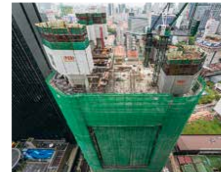
For the RCS enclosure, different materials can be used, e.g. LPS mesh panels, trapezoidal sheeting, multi-layer wooden boards or netting.
