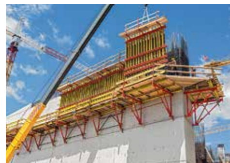
CB Climbing Brackets served as a platform system for the VARIO Wall Formwork.
