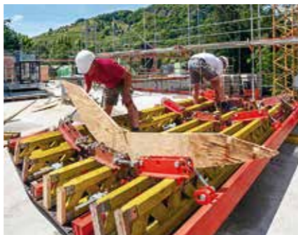
The self-cleaning adjusting spindles are adjusted to fit the required curvature by means of a ratchet spanner.
