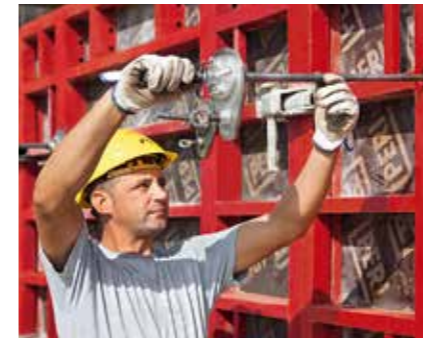
The specially-developed MX Tie is installed from one side only and is used without spacer tubes and cones. This means material and working time savings.
