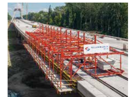
With the VARIOKIT Cantilevered Parapet Carriage, the horizontal loads are completely transferred via friction; anchoring is not required.
