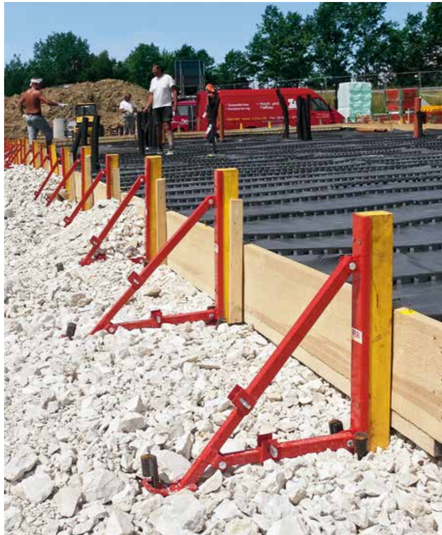
For forming bottom slabs up to 60 cm thick, the Stopend Trestle is used; it is easily aligned by means of the adjustable strut and integrated clamping wedge.
