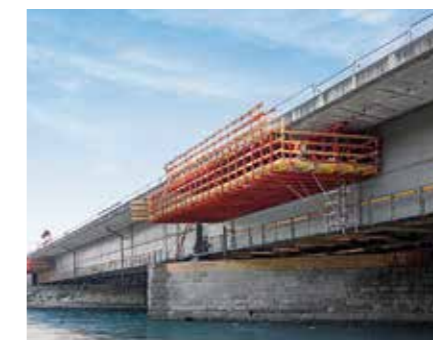
The Cantilevered Parapet Track is secured to the underside of the bridge by means of rails and rollers. The bridge is freely accessible; the flow of traffic remains unaffected.
