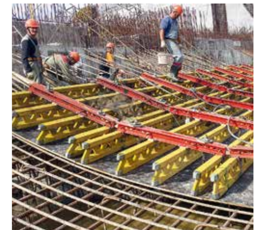
PERI planned and delivered customized solutions for the complex building geometries.
