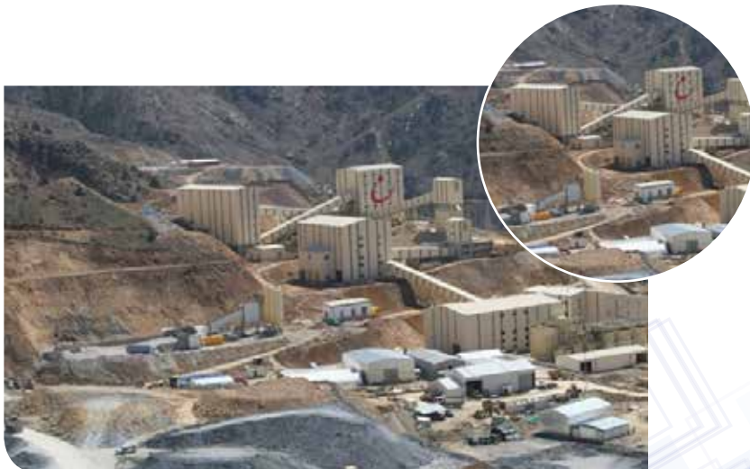
-Roller Compacted Concrete (RCC) Plant Installation for dam projects
