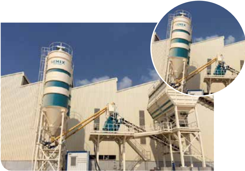
-Concrete Batching Plant Installation for the production of Ductile Iron Pipe
