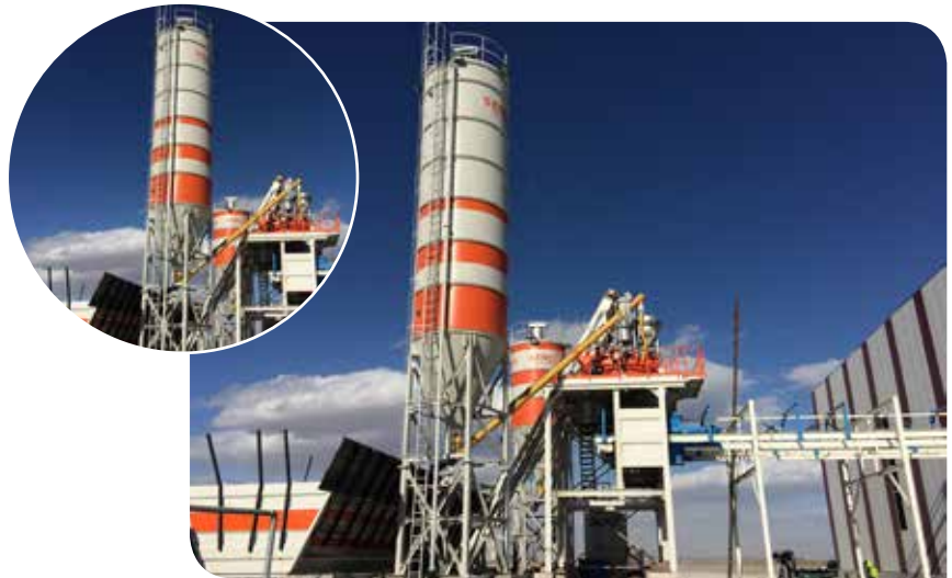
-Concrete Batching Plant Installation for precast production
